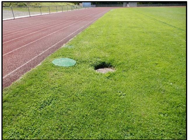
Photo 6 – Typical area drain in field
